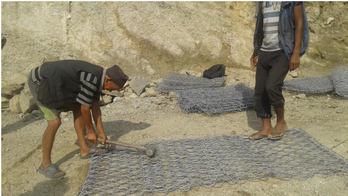
Photo 3: Gabion wire basket assembling in Bajura
