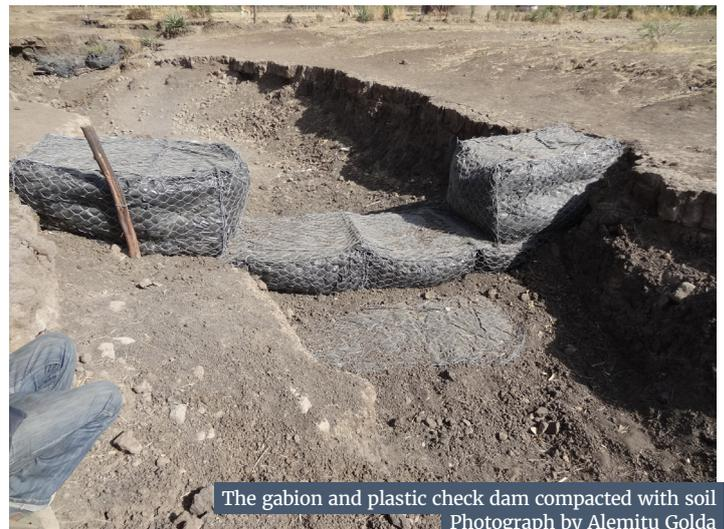
The gabion and plastic check dam compacted with soil
